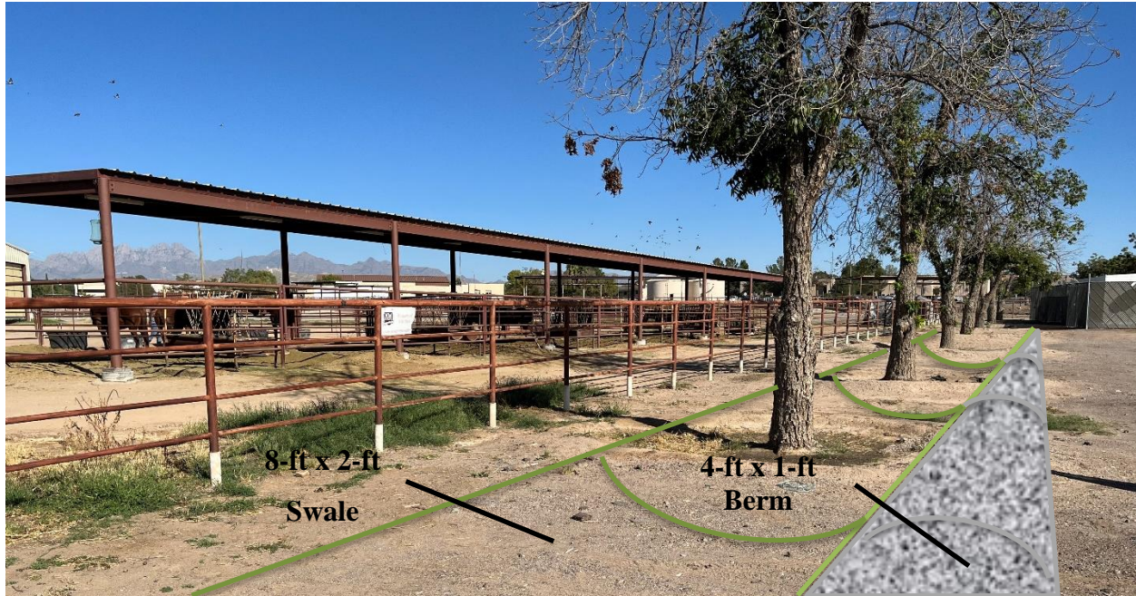
FIGURE 8-14: CORRALS RUNOFF MITIGATION
