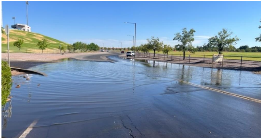
FIGURE 5-4: PONDING AT ARROWHEAD AND WELLS
