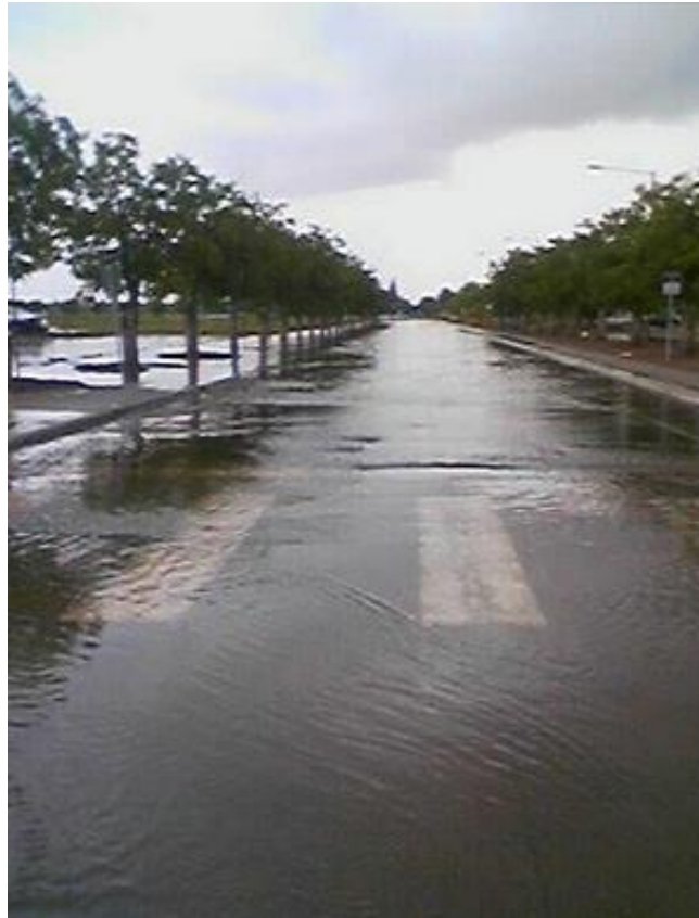
FIGURE 5-3: FLOODING ON COLLEGE DR (2007)
